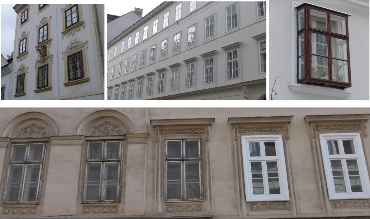
Fig 3. Beautiful casement windows (upper row) versus inconsistent appearance of a façade with casement windows of little maintenance and incongruous replacements by multi-layer insulation-glass windows made of plastic (© P. Schober).
